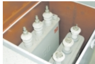
The Used Equipment Containing PCB in Storage Box (Mishima Olympus Co., Ltd.)
