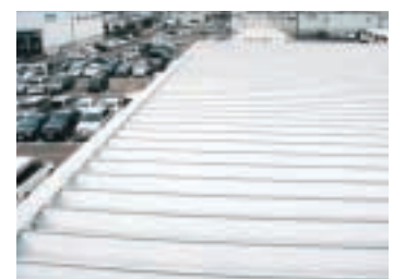
Insulation is placed on the Roof of Cleaning Room
