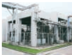
Renovation of Public Nuisance Treatment Facilities
