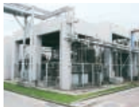
Renovation of Public Nuisance Treatment Facilities
