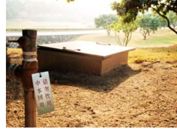
Water recycling facilities
