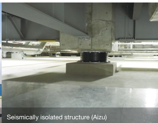
Seismically isolated structure (Aizu)
