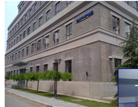
Training Center in Beijing City
