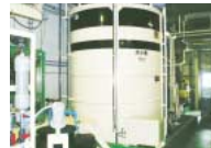
Relocation of raw water tank on the ground
