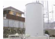
Relocation of kerosene tanks on the ground
