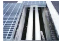
Relocations of wastewater piping on the ground
