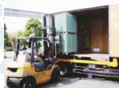
Loading of waste materials on containers
