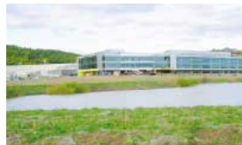
The Olympus corporate headquarters was located so as not to disturb any wetlands.
