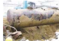
Removal of underground tanks
